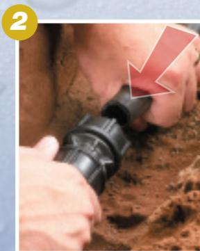
2 Ensure 2 threads are showing and simply slide the pipe in until the first point of resistance is felt.
