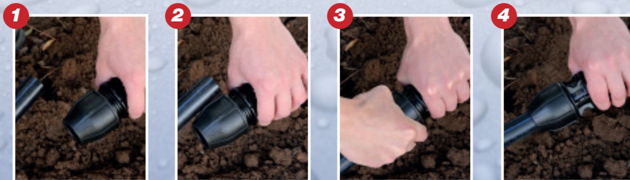
1 Cut the pipe square. There is no need to chamfer or lubricate the pipe. Ensure 3 threads are showing.
