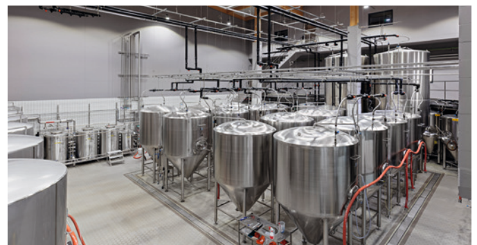
The pipe cooling system was installed up to the tanks.
