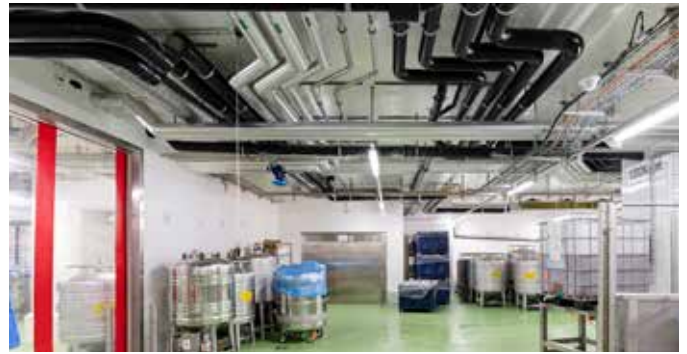
The modernization involved a stretch of around 150 meters of the system.
