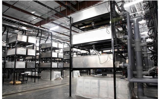
Rhodium uses immersion cooling, fully submerging their servers to achieve maximum efficiency.
