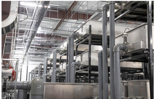
ChlorFIT, made with Corzan® CPVC, is a highly robust and corrosion resistant Schedule 80 piping system offering superior reliability and long-lasting performance in commercial and industrial applications.
