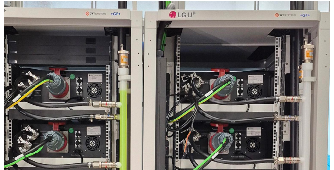
Polymer manifolds are custom-engineered based on the project requirement and rack densities.
