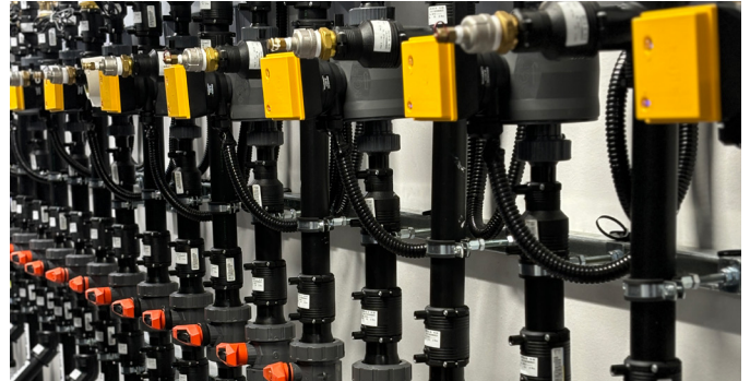
The manifold wall at STDCT plays a key role in optimizing flow for direct-to-chip (D2C) liquid cooling by ensuring balanced, efficient, and easily monitored coolant distribution.
