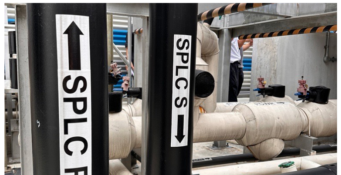
Ensuring stable temperatures for the chilled water lines with pre-insulated PE piping system COOL-FIT
